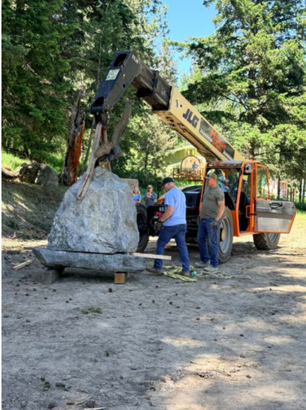
Post 4042 working on the monument.
