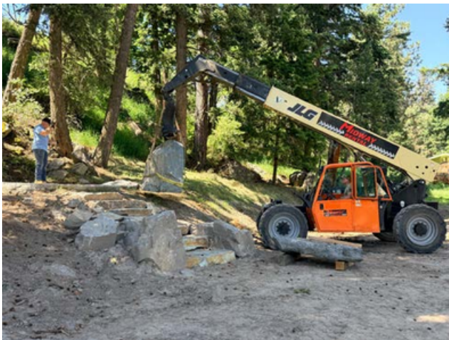
Post 4042 moving rock into place for the monument.
